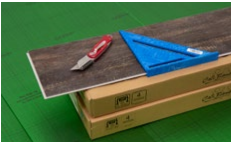
Cutting boards using Score and Snap technique
