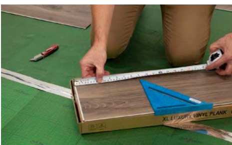
Cutting boards using Score and Snap technique
