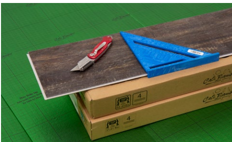
Cutting boards using Score and Snap technique
